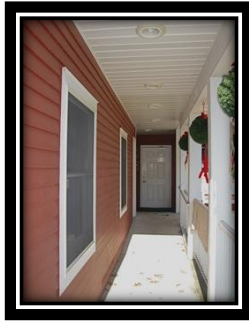
View on walkway
